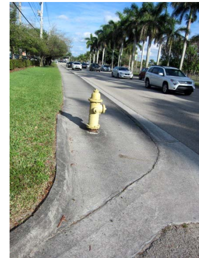
Observed sidewalk obstructions include utility poles in the middle of the sidewalk, with additional cables blocking the path for an alternate route (Top Left, Image source – Google Earth), Utility boxes and fire hydrants in sidewalks (Top Right), traffic signs (Bottom Left), and fire hydrants in sidewalks at curb areas (Bottom Right), all of which present issues for pedestrians, and some of which are non ADA compliant.
